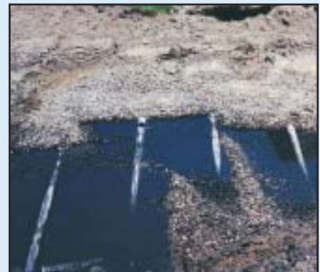
A failed system exposed.
