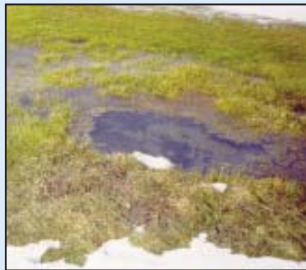
Effluent pond on top of the leaching bed.
